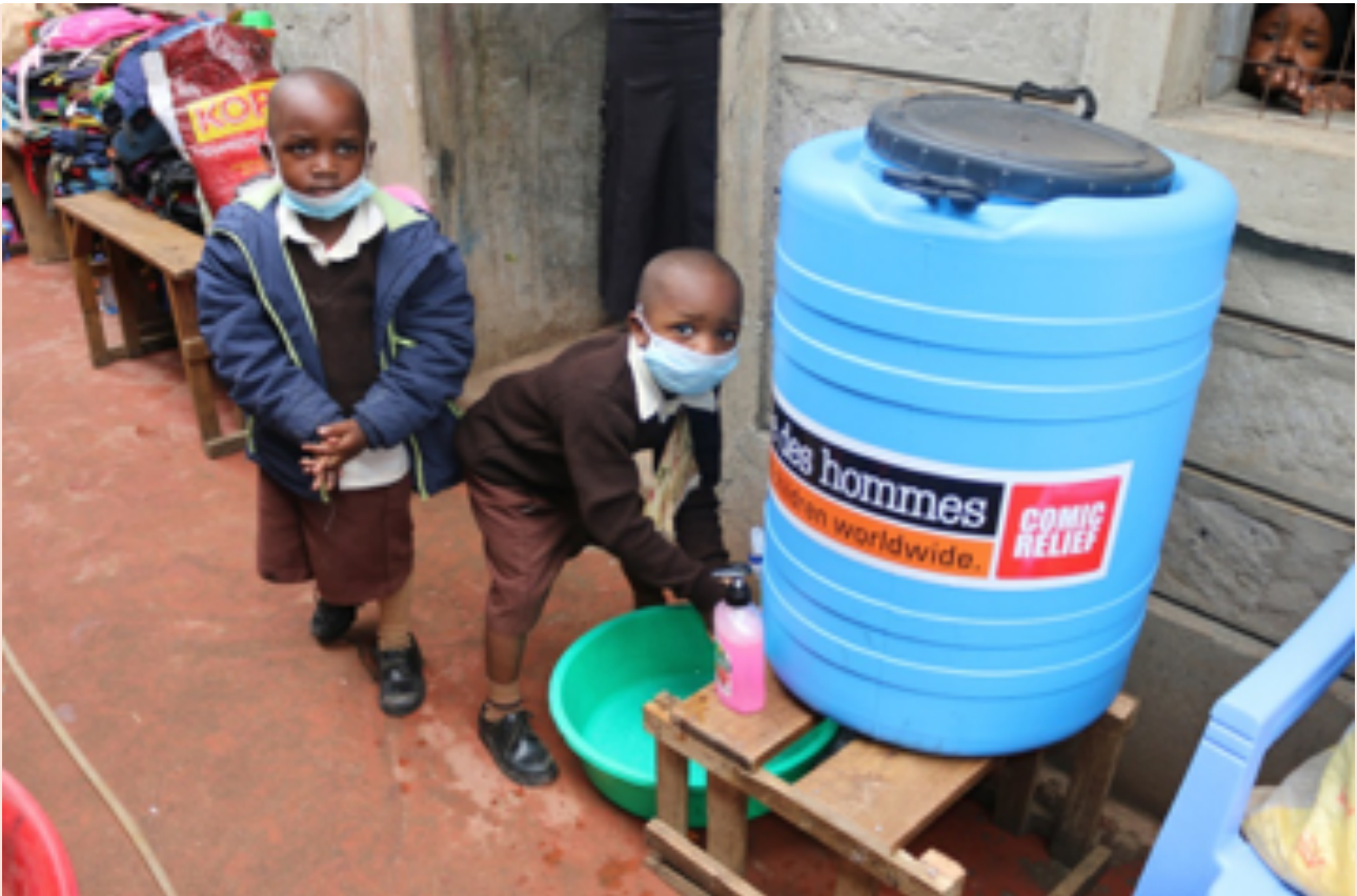
Photo 1: ECD centres were provided with water, sanitation and health (WASH) facilities
